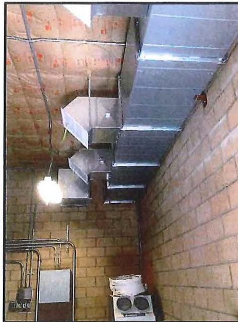
Installed ceiling insulation and AC air ducting
